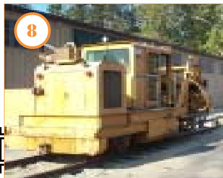
8 July: A crew from Sharp & Fellows Co. machine-tamps the ballast and surfaces the track, bringing it to the final level and alignment. The large yellow machine does the tamping; the rest of the work is done by hand.
