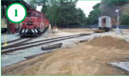
Waiting for landscaping! The open area to the south of the new Locomotive Pavilion was formerly the site of the volunteer Restoration Yard. Seen here in the early days of the project, the area has been cleared to make way for the new BBQ and Picnic area.
