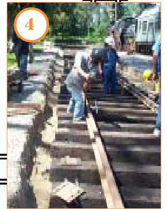
4 April 9: Rails are laid out, bolted together and spiked down by volunteers.
