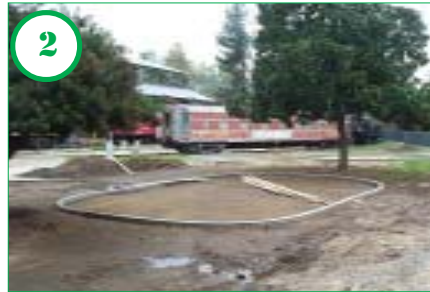
One of the new "BBQ Rings" is taking shape.
