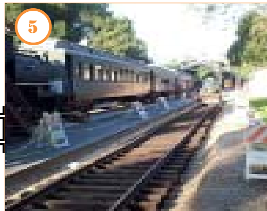
5 April 16: The freshly-laid track is now ready for ballast.
