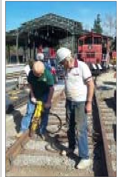
Roger's favorite work is on the track. Here he explains the finer points of pneumatic spike-driving to fellow volunteer Greg Hewlett.
