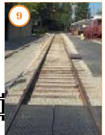
9 August 1: The completed Track 5-West is now ready and waiting for its cadre of historic locomotives and cars to be moved into display position.
